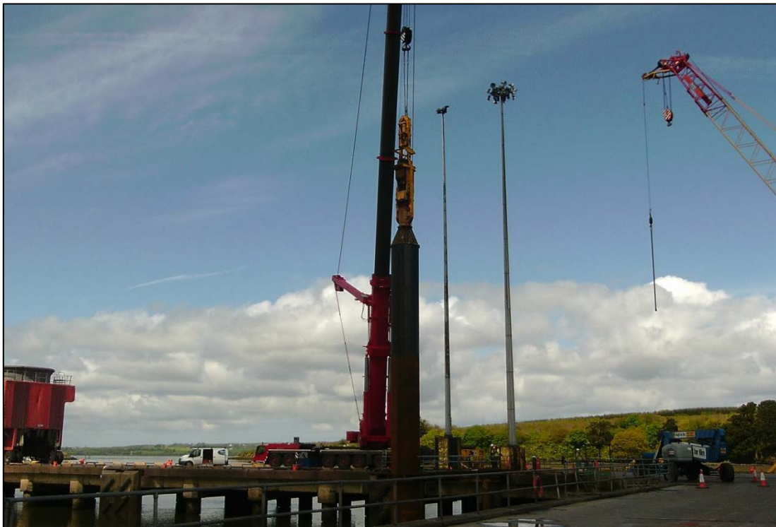
Plate 2.3 Piling Hammer in Use for Tubular Pile Installation
