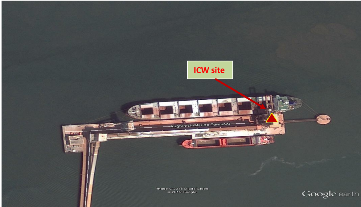
Figure 3: Rusal Aughinish jetty
