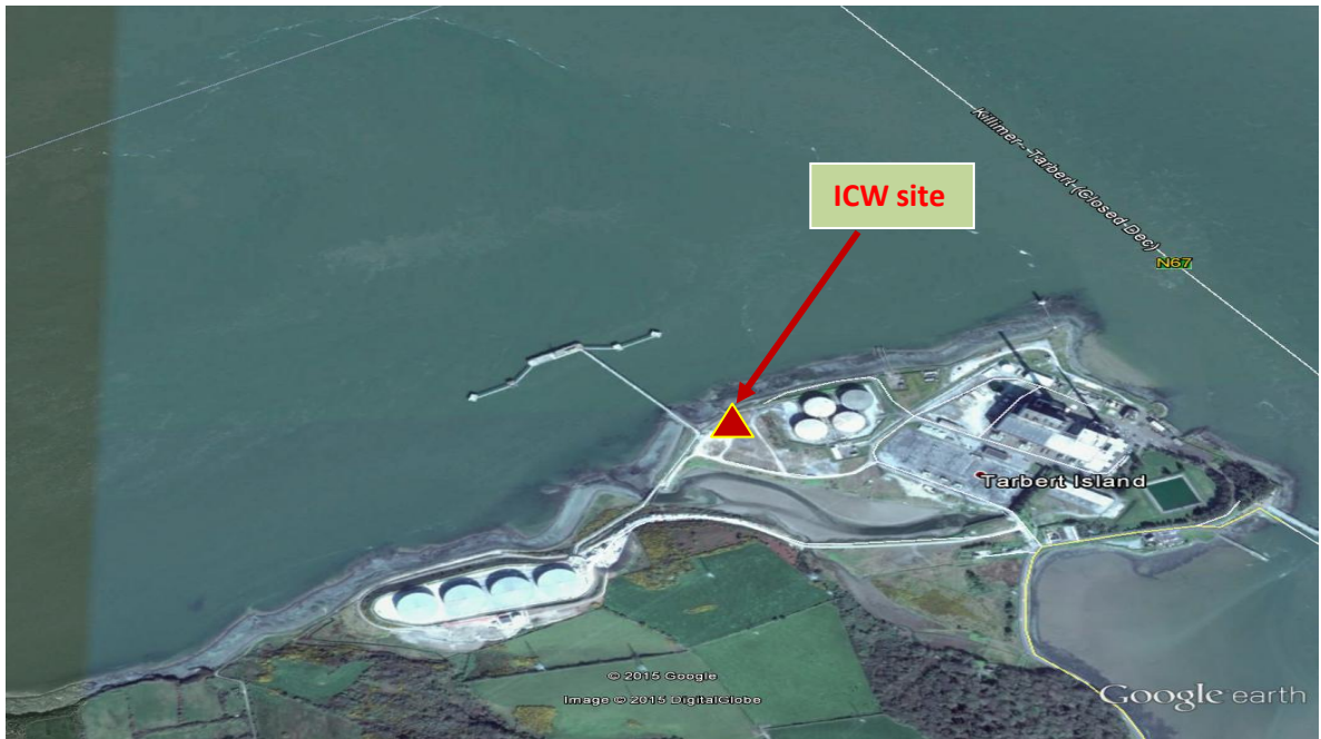
Figure 5: Tarbert Oil Jetty.
